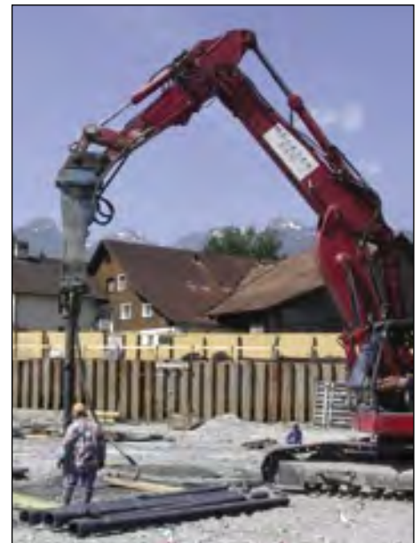
Excavator and hammer for pile installation
