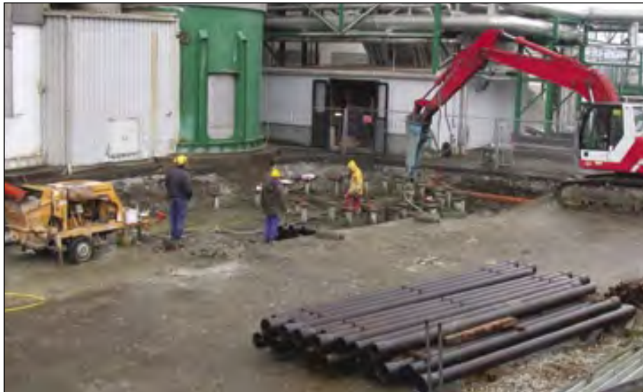
Grout injection through the pile bore during driving
