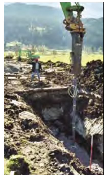
Banksman and staff for driving alignment
