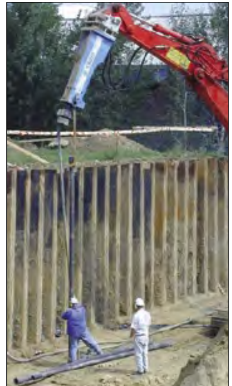
Pitching of a pile (note: lifting sling, shackled at the nose of the hammer)
