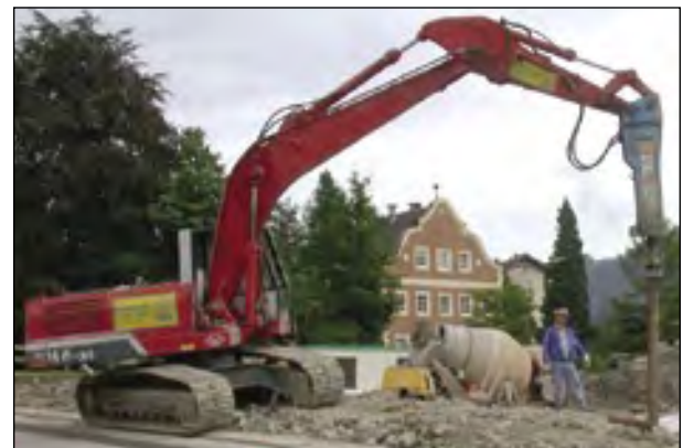
Driven Piles (end-bearing) for apartment blocks
