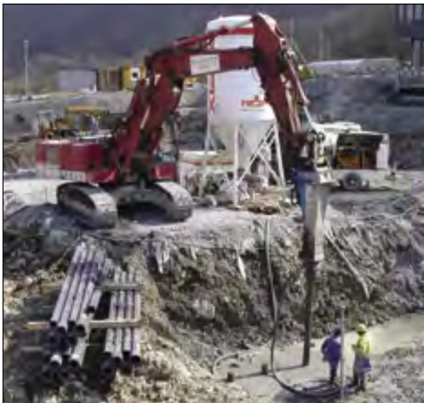
Grout injection piles for a factory unit
