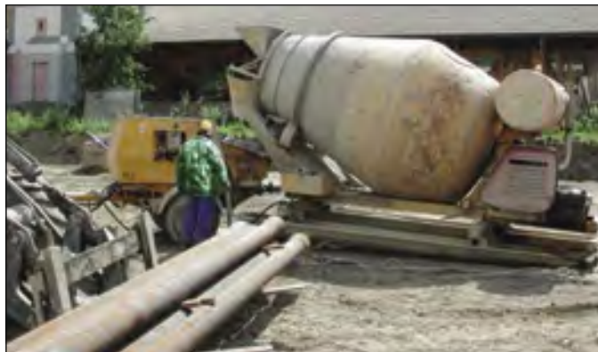
Concrete pump and agitator for grout injection driven piles (pump performance: 20 Ltr / hr, 20-40 bar)
