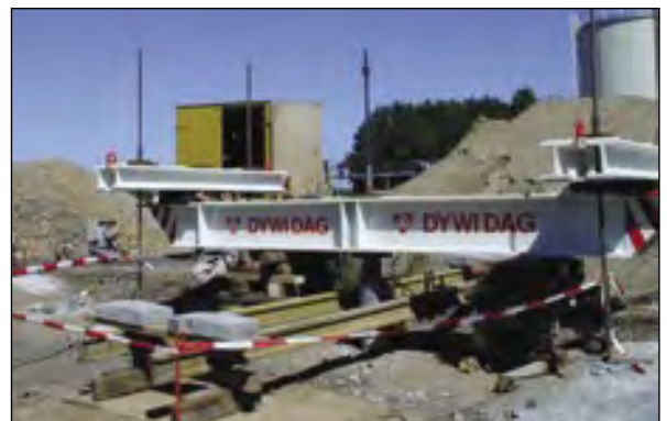
Static pile test
