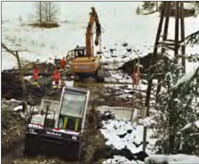
Piles for power transmission towers
