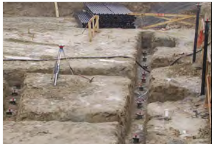
Ductile Iron Piles driven at formation level of ground beams
