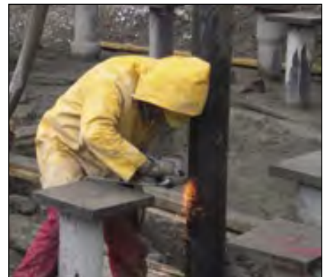
Simple cut down of pile head using a disc cutter
