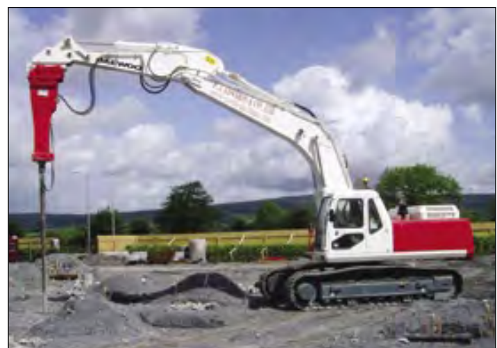
Installation of Ductile Iron Piles for new housing development and hotel
