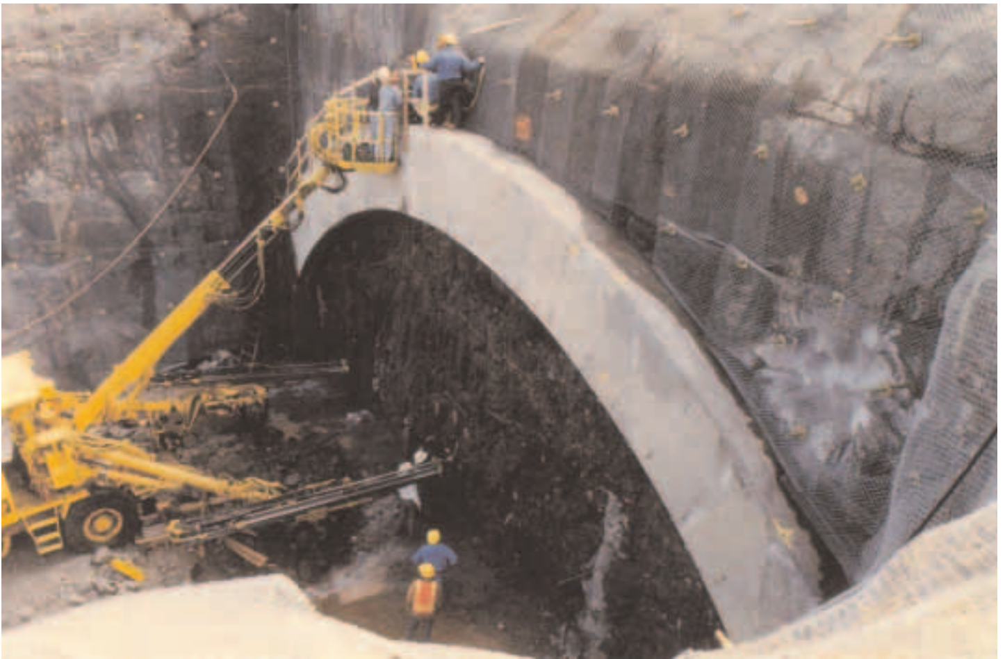
Lafayette Bluff Tunnel, U.S. Highway 61, Minnesota
