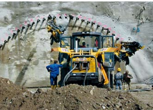
Cross-section pipe umbrella support system
