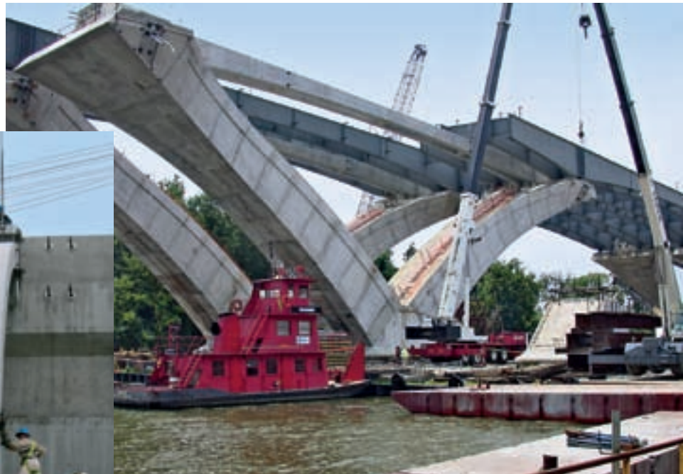
Woodrow Wilson Bridge, Washington, D.C., USA
